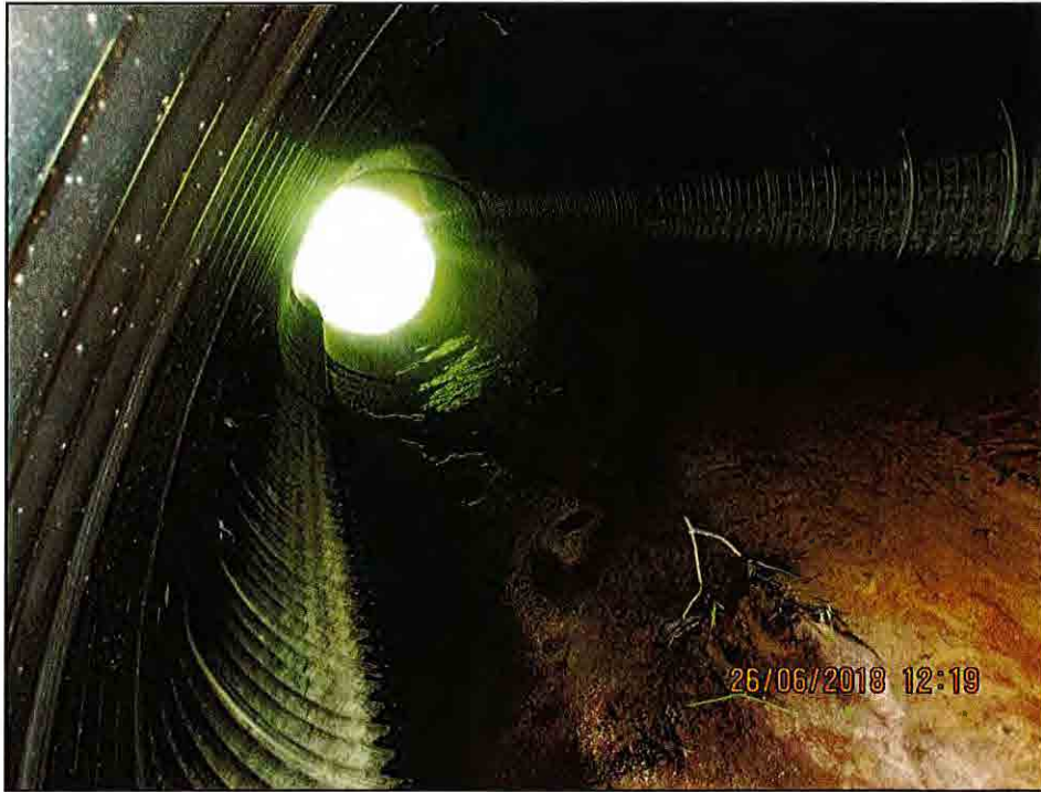
Barrel looking West
