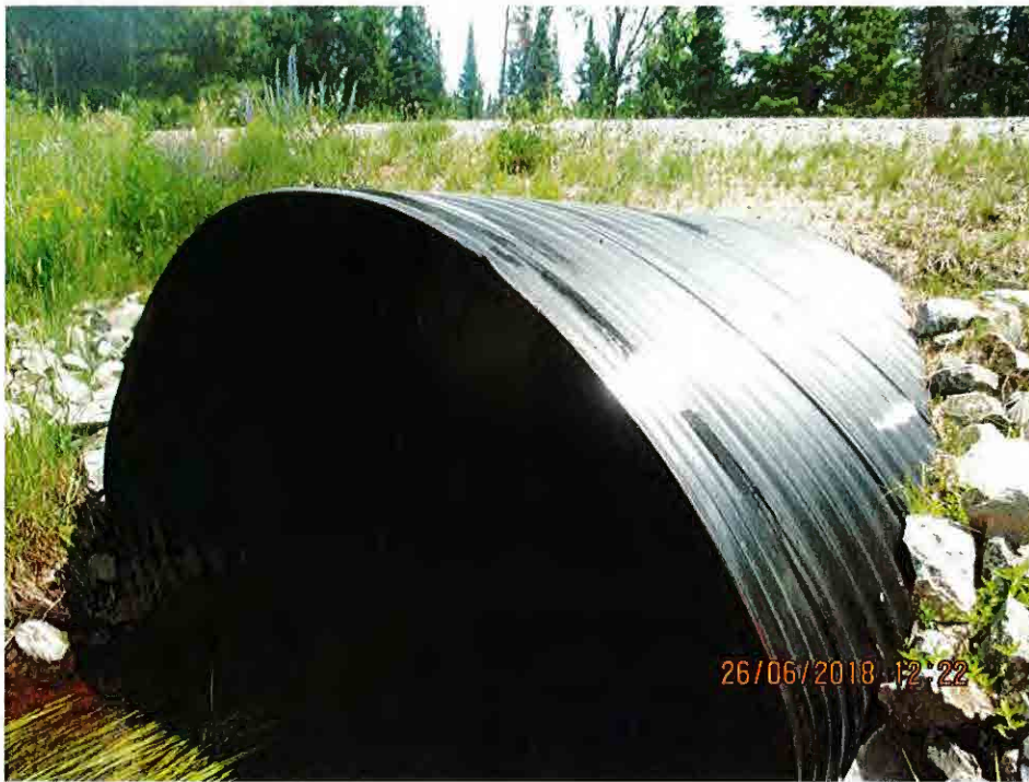
Inlet (West end)
