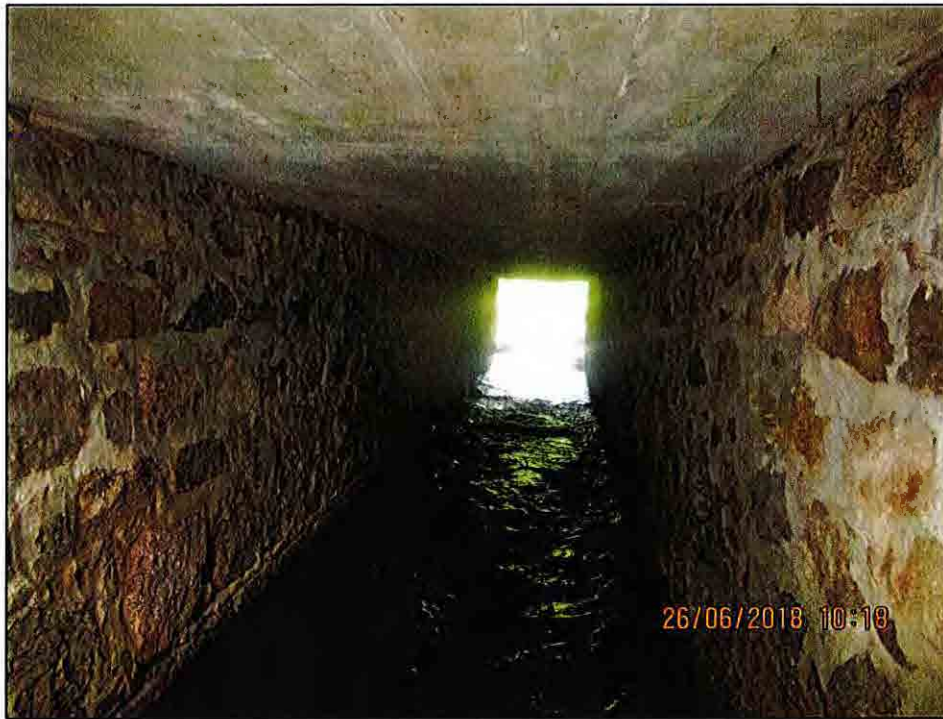
Barrel looking West
