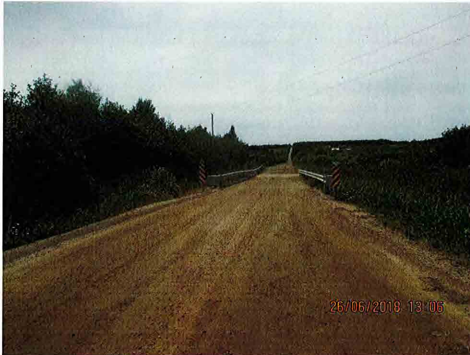
Roadway looking West
