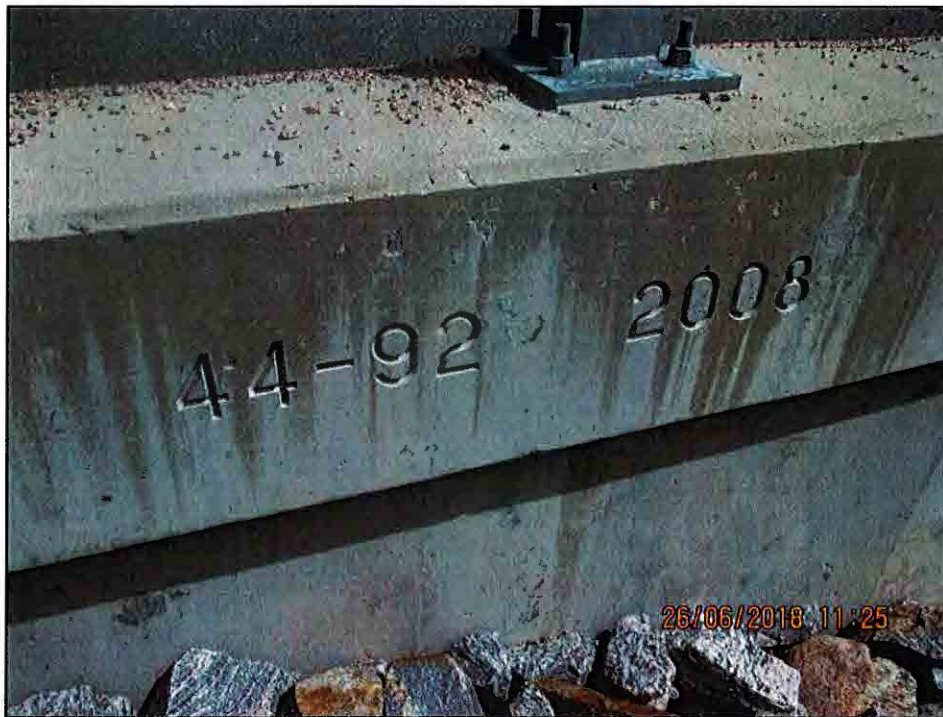
Southwest wing wall
