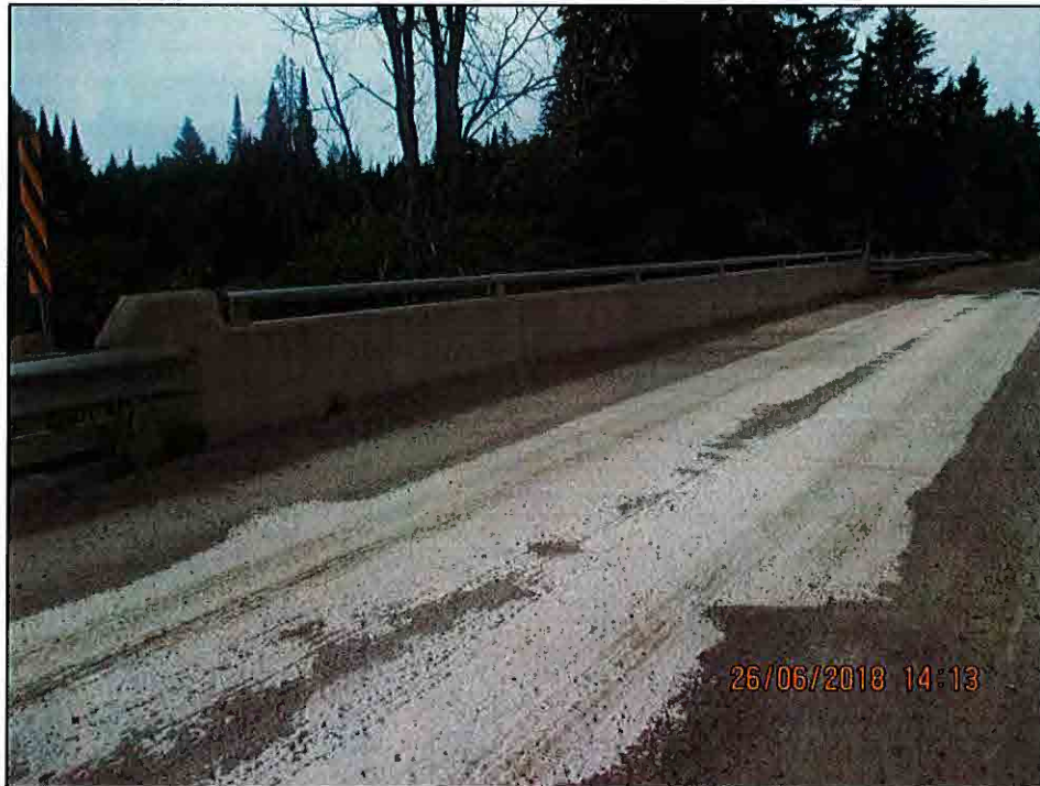
West parapet wall
