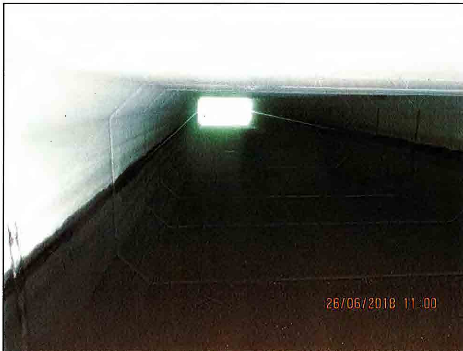
Barrel looking South
