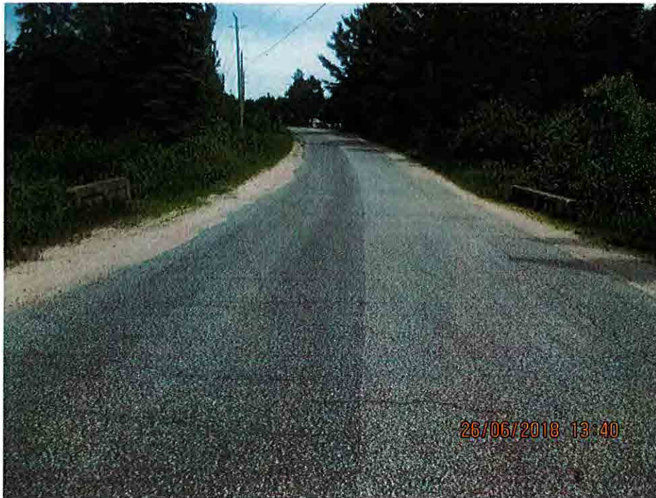
Roadway looking East
