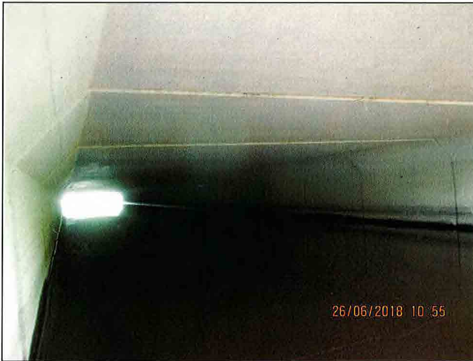
Barrel looking South
