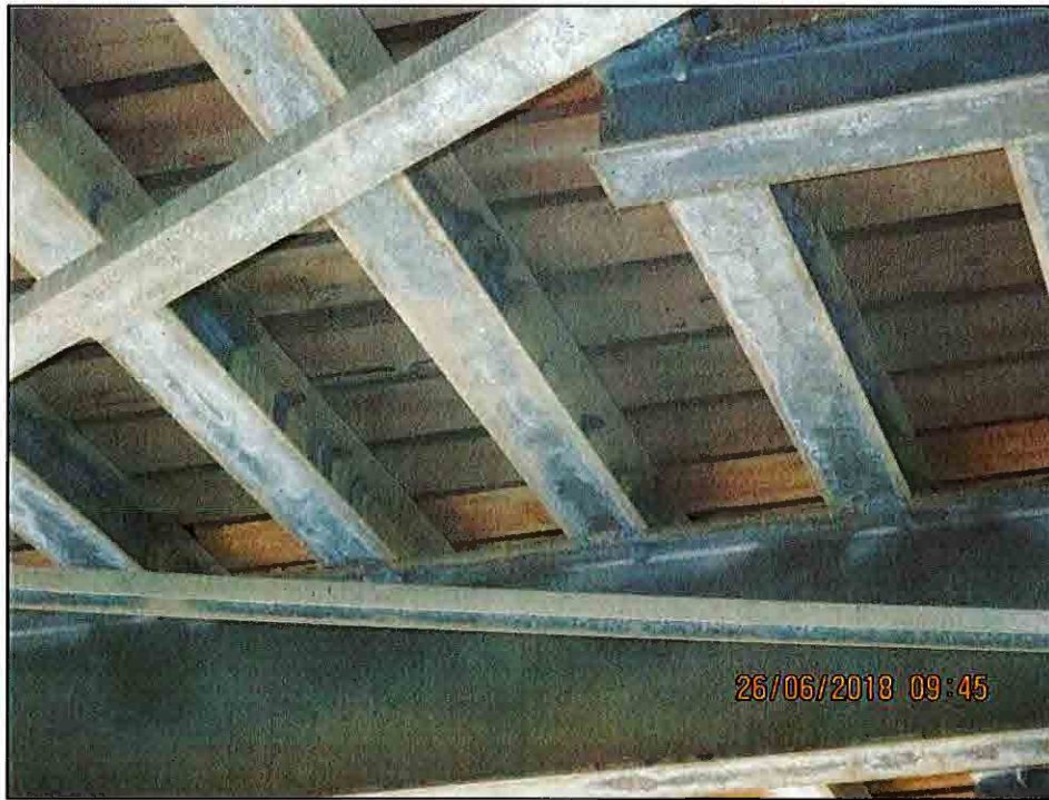
Split soffit timbers
