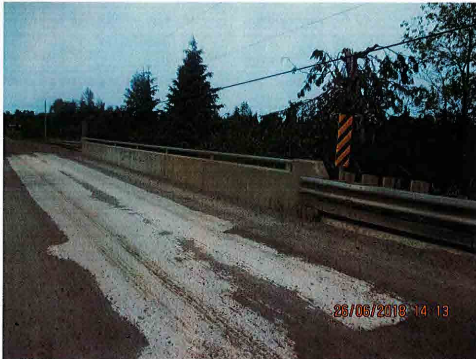
East parapet wall
