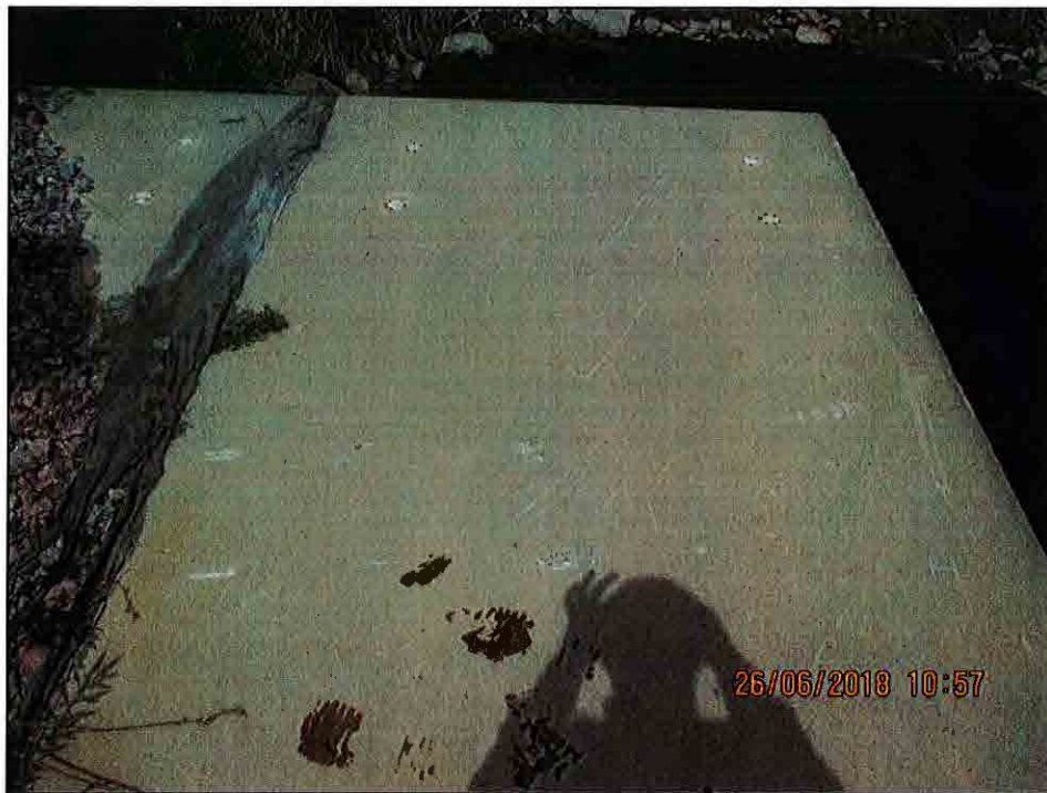
Top of culvert at North end
