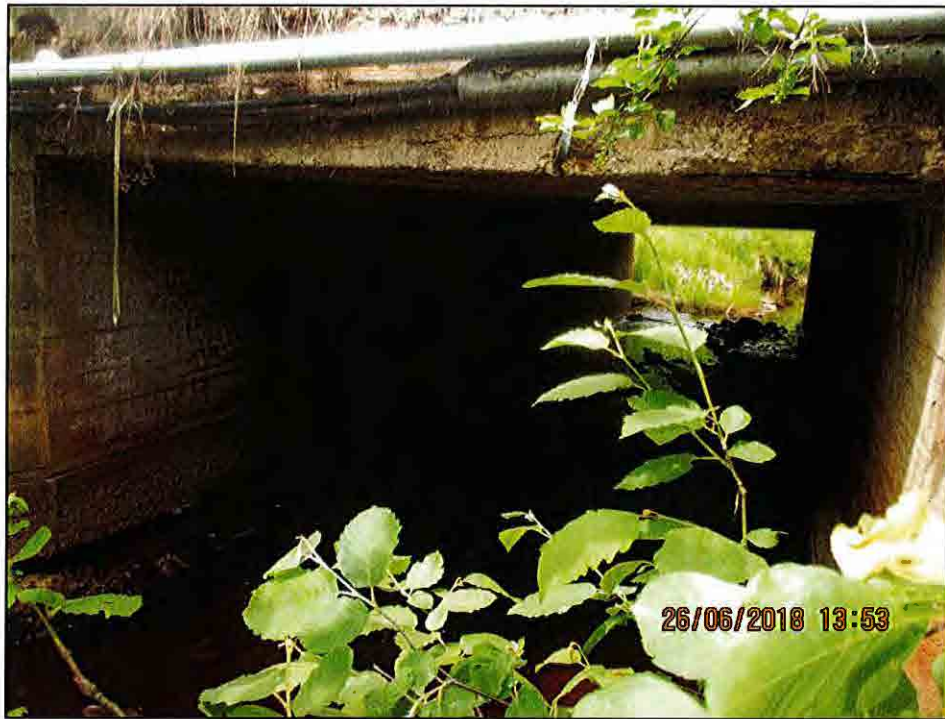
Outlet (South end)
