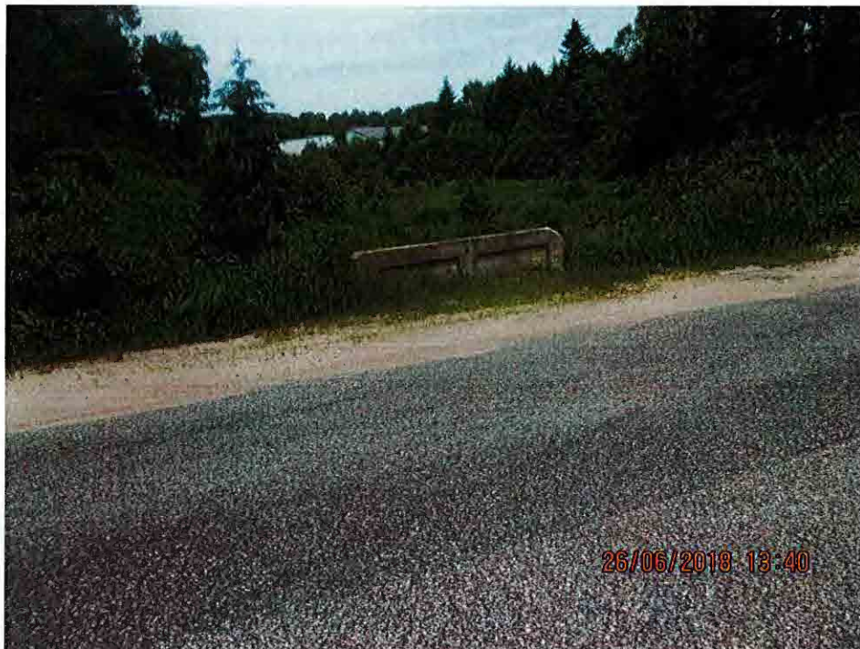
North barrier wall
