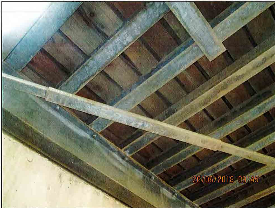
Split soffit timbers
