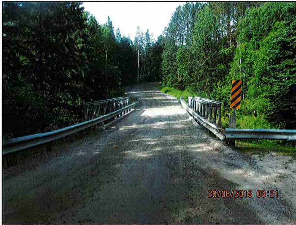
Roadway looking West
