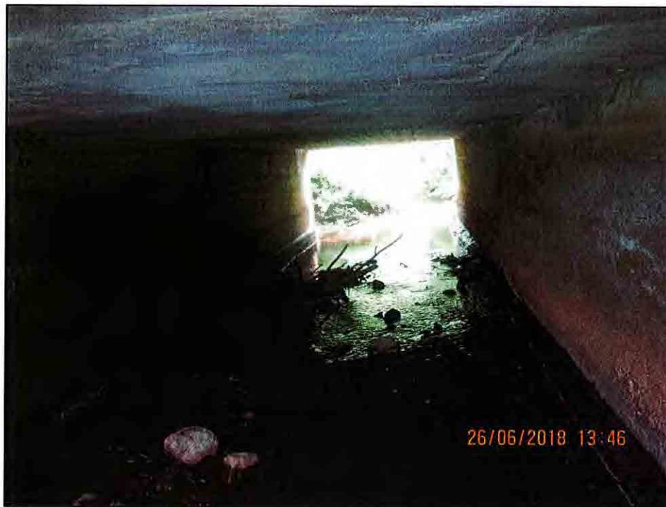
Barrel looking South
