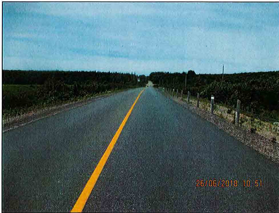
Roadway Looking West
