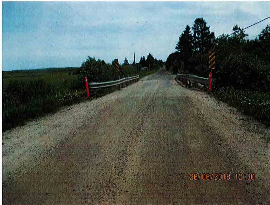
Roadway looking East
