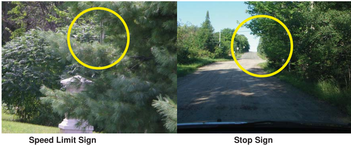
Figure 15 Obscured Regulatory Signage
