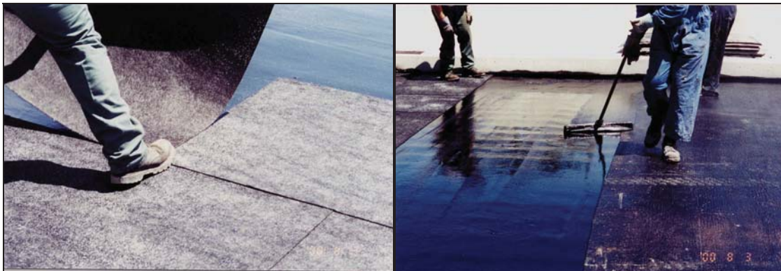
Figure 17 Bridge Deck Maintenance
