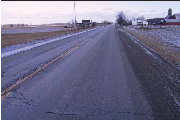
Figure 2 "1 to 5" Year Need Road (Resurfacing)
