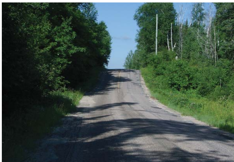
Figure 11 Substandard Vertical Alignment
