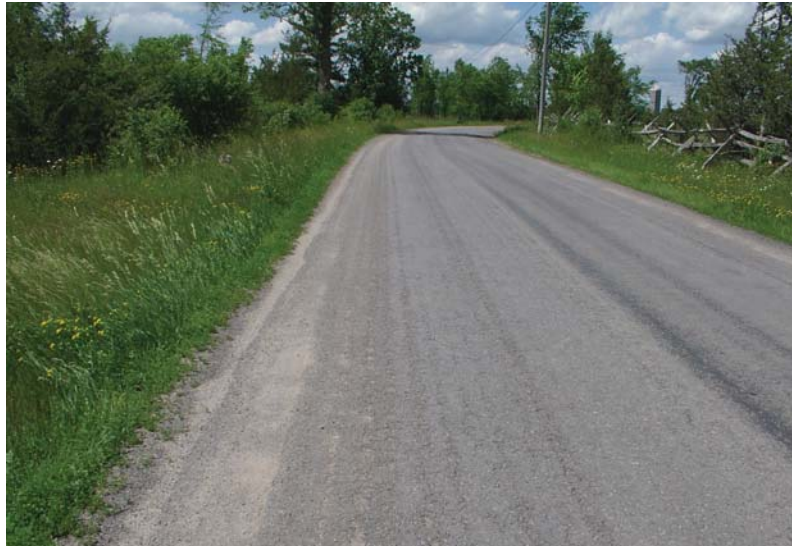
Figure 12 Substandard Horizontal Alignment
