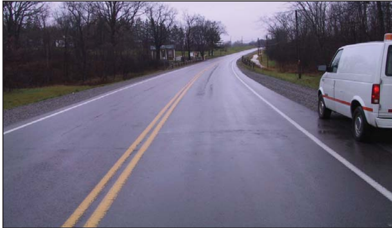
Figure 4 "Adequate" Road (Approx. 7 year old)
