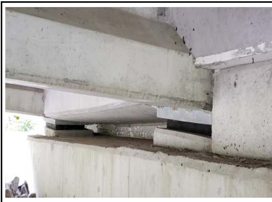
Photo 10 Bearing pad at west abutment wall
