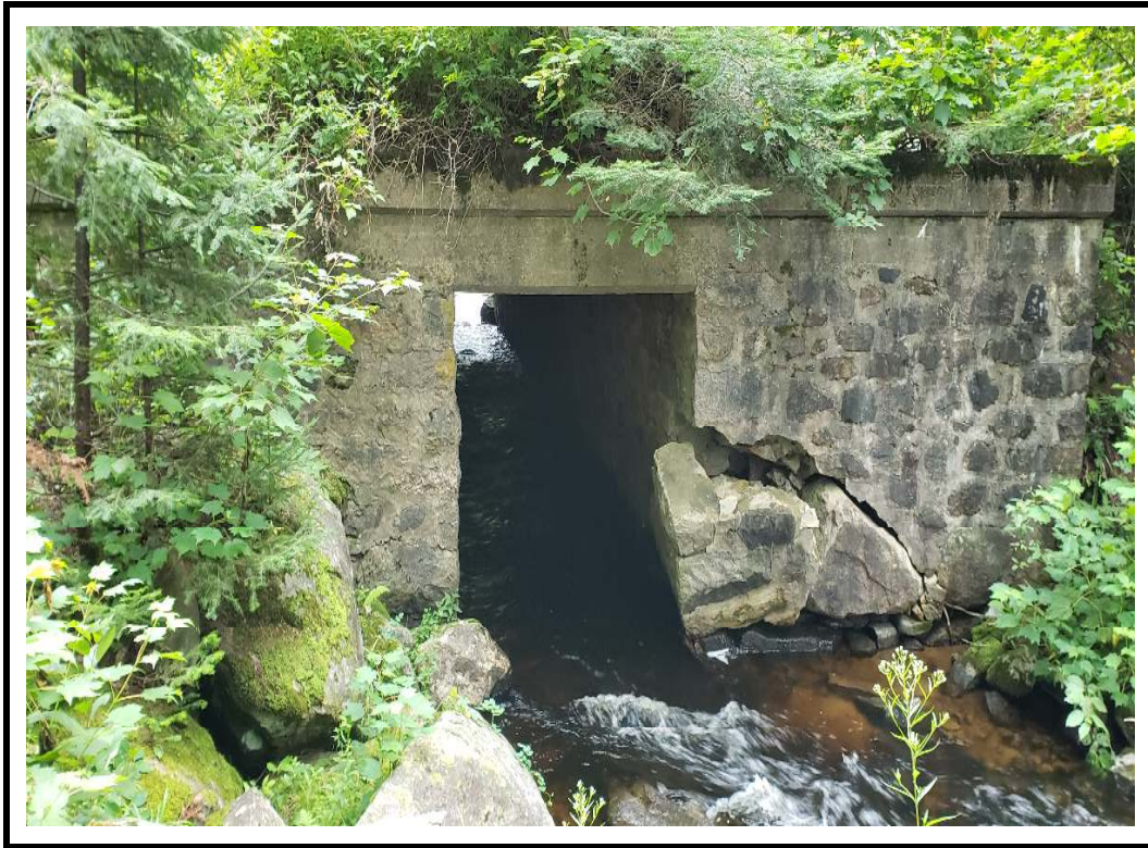
Photo 5 East elevation (prior to 2020 rehabilitation)
