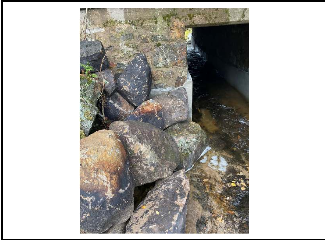
Photo 17 Northwest wingwall (after 2020 rehabilitation)
