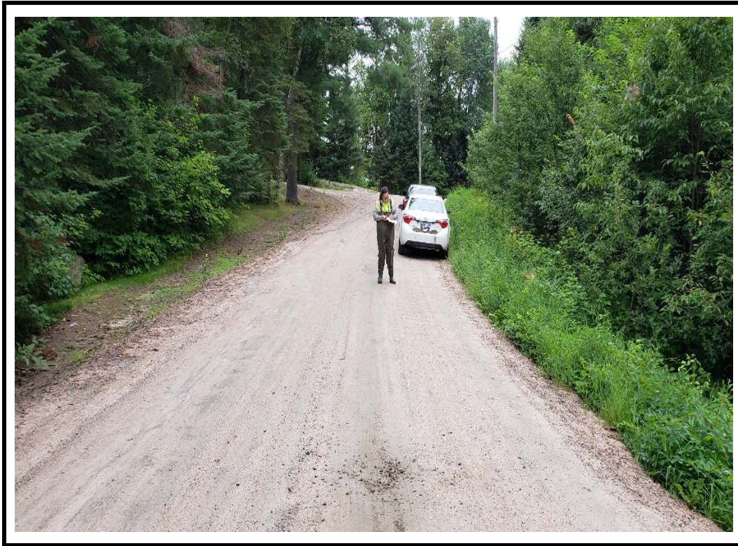
Photo 3 North approach from centre of structure
