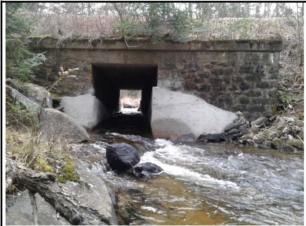
Photo 14 East Elevation (after 2020 rehabilitation)
