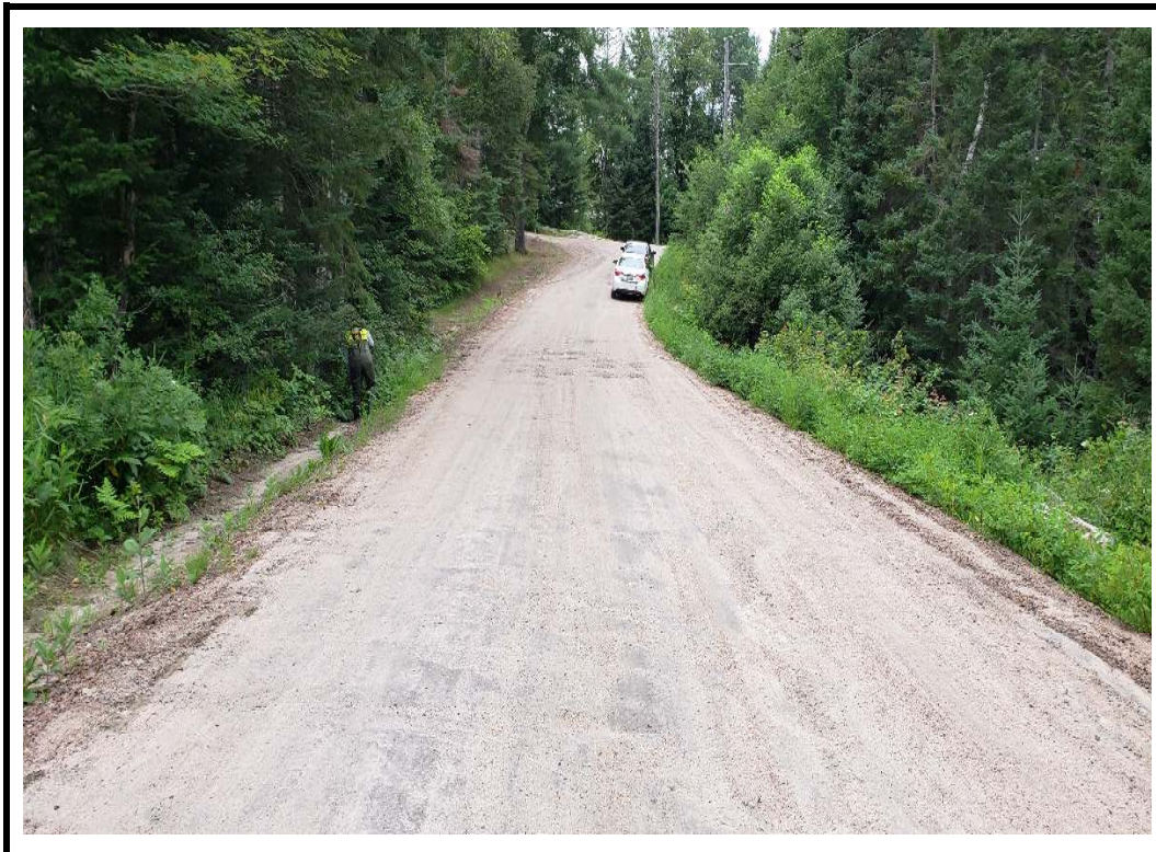
Photo 2 Structure from south approach
