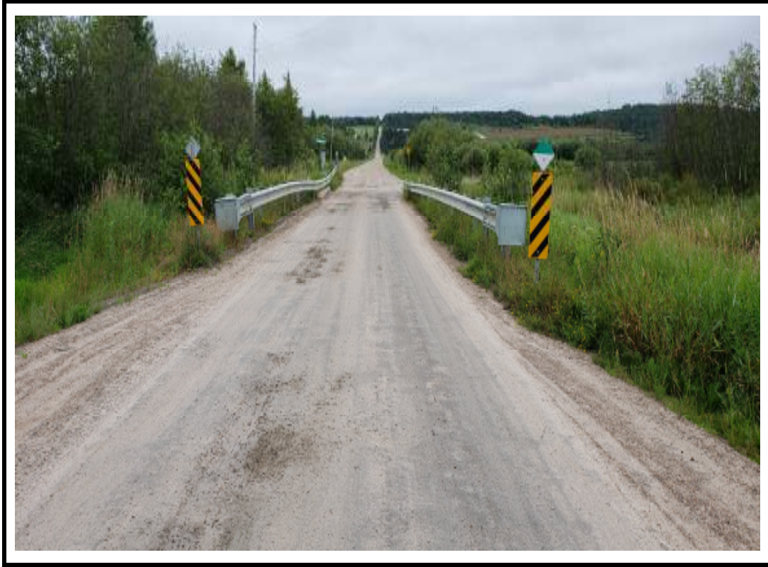
Photo 1 Structure from east approach
