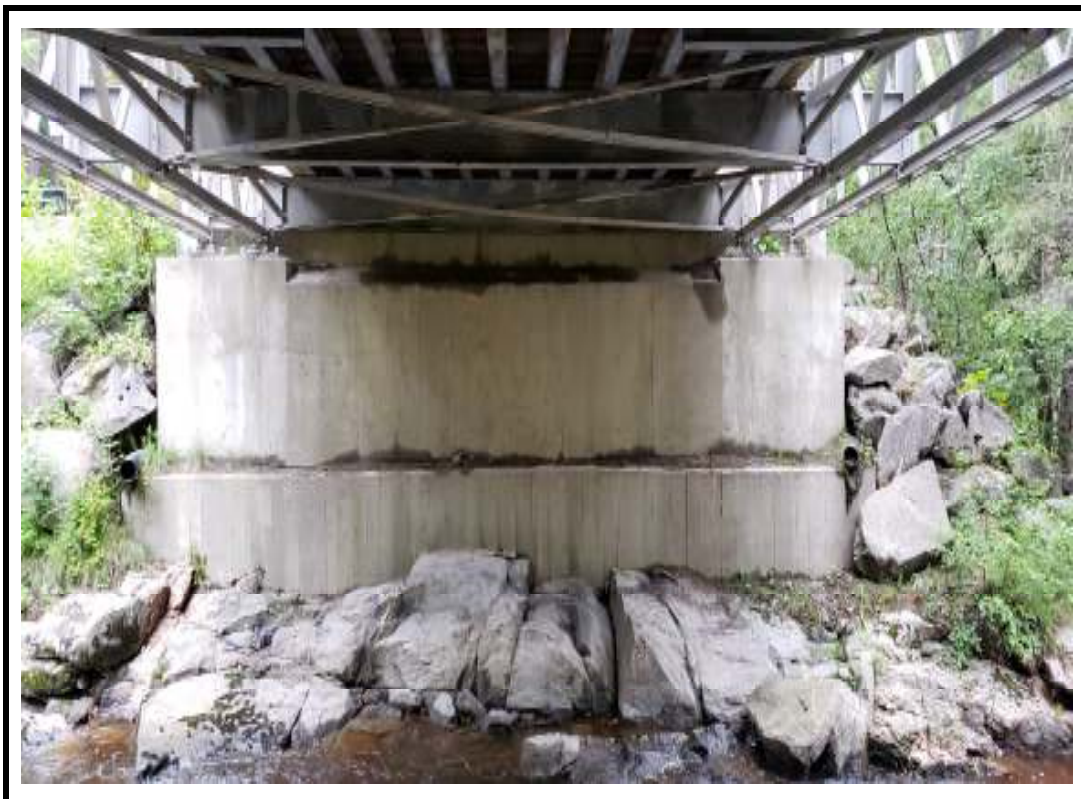
Photo 16 East abutment wall
