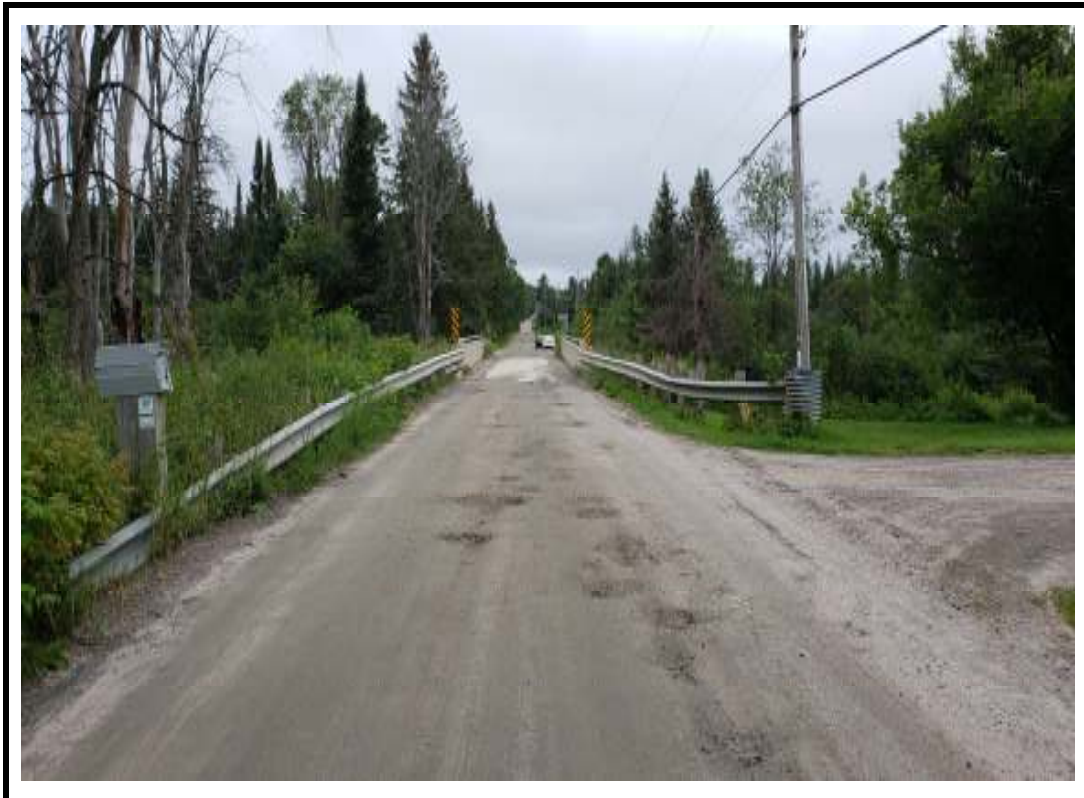
Photo 2 Structure from south approach
