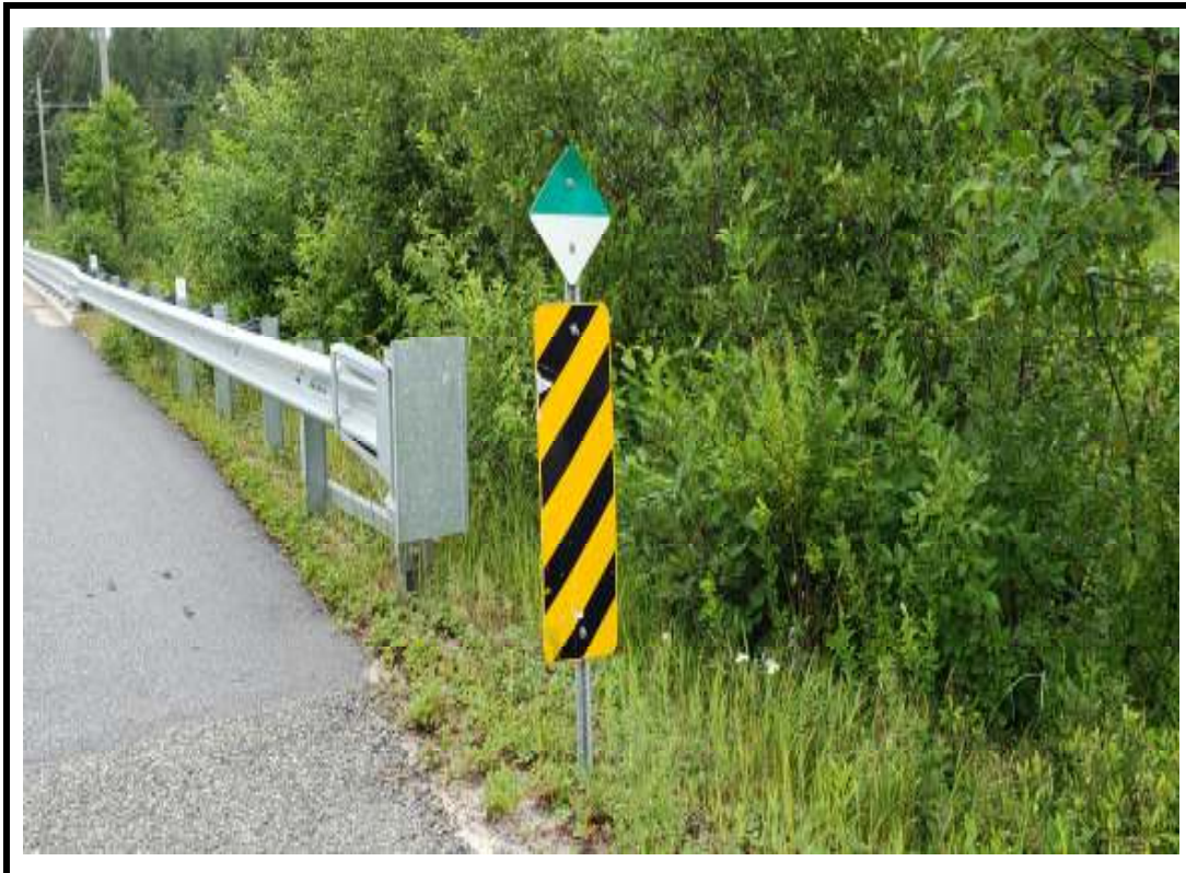
Photo 8 Small dents and abrasion noted on southeast hazard sign
