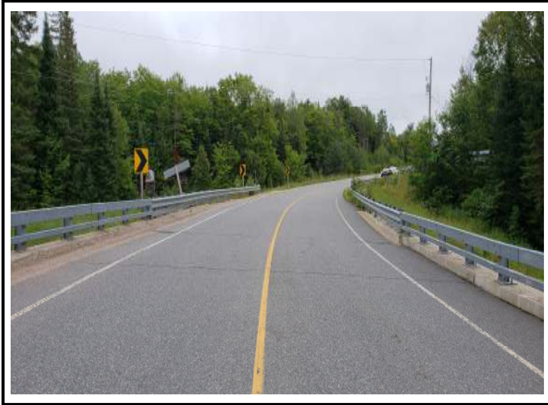
Photo 3 East approach from centre of structure
