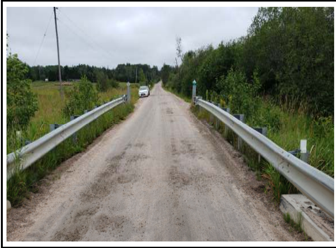
Photo 3 East approach from centre of structure
