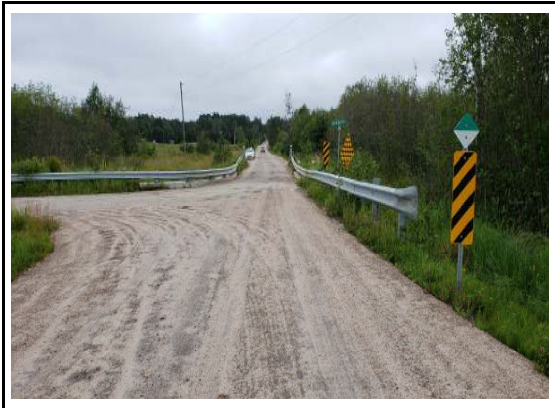
Photo 2 Structure from west approach
