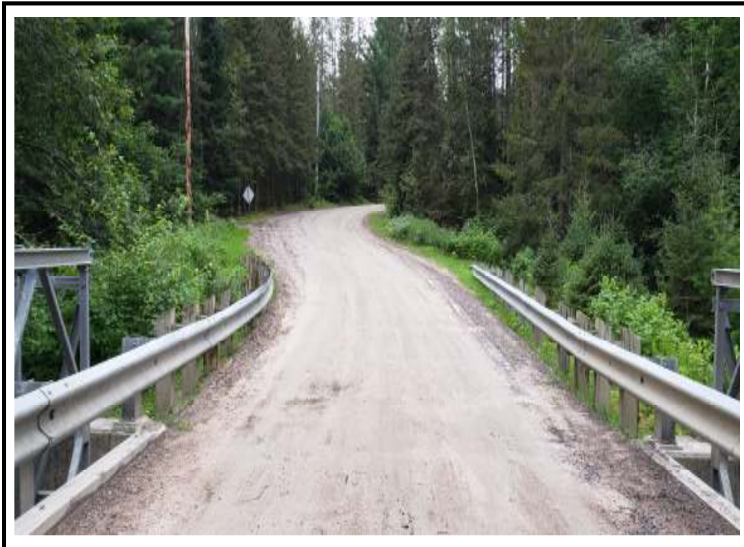
Photo 4 West approach from centre of structure
