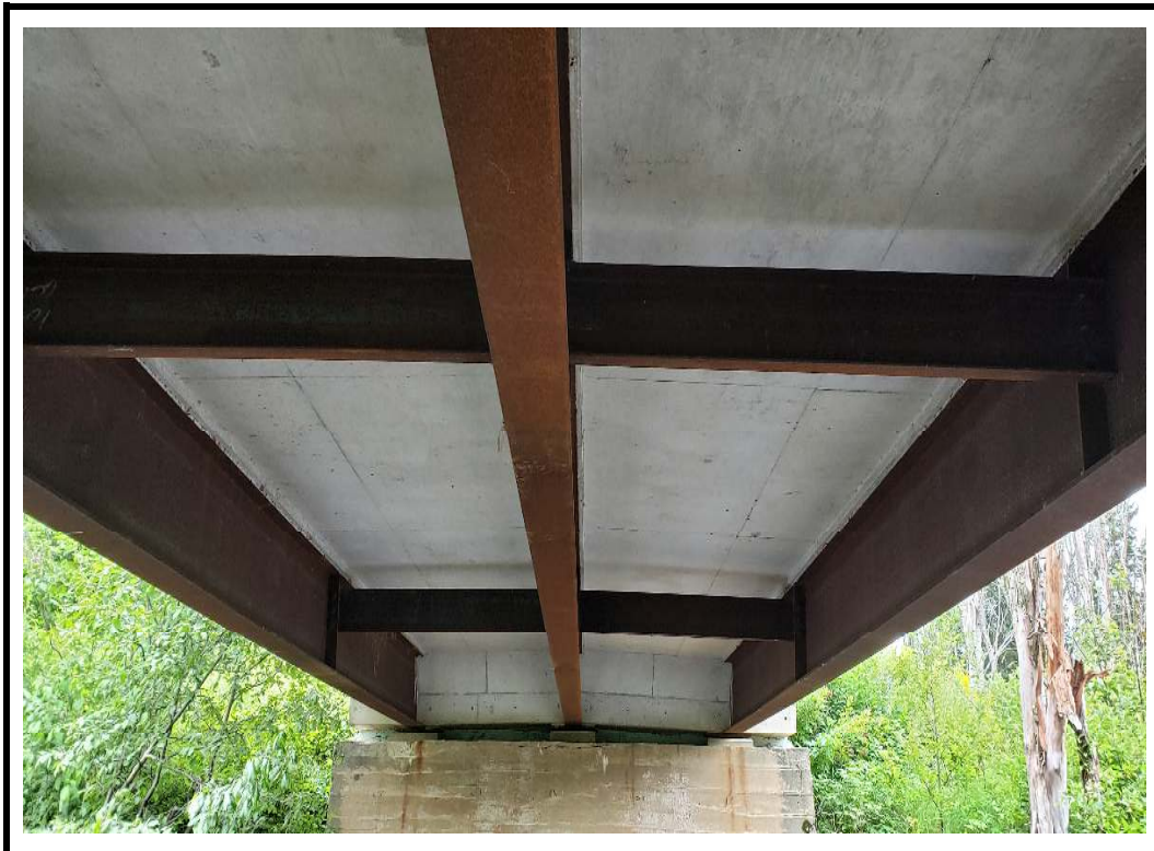
Photo 12 West underside of structure
