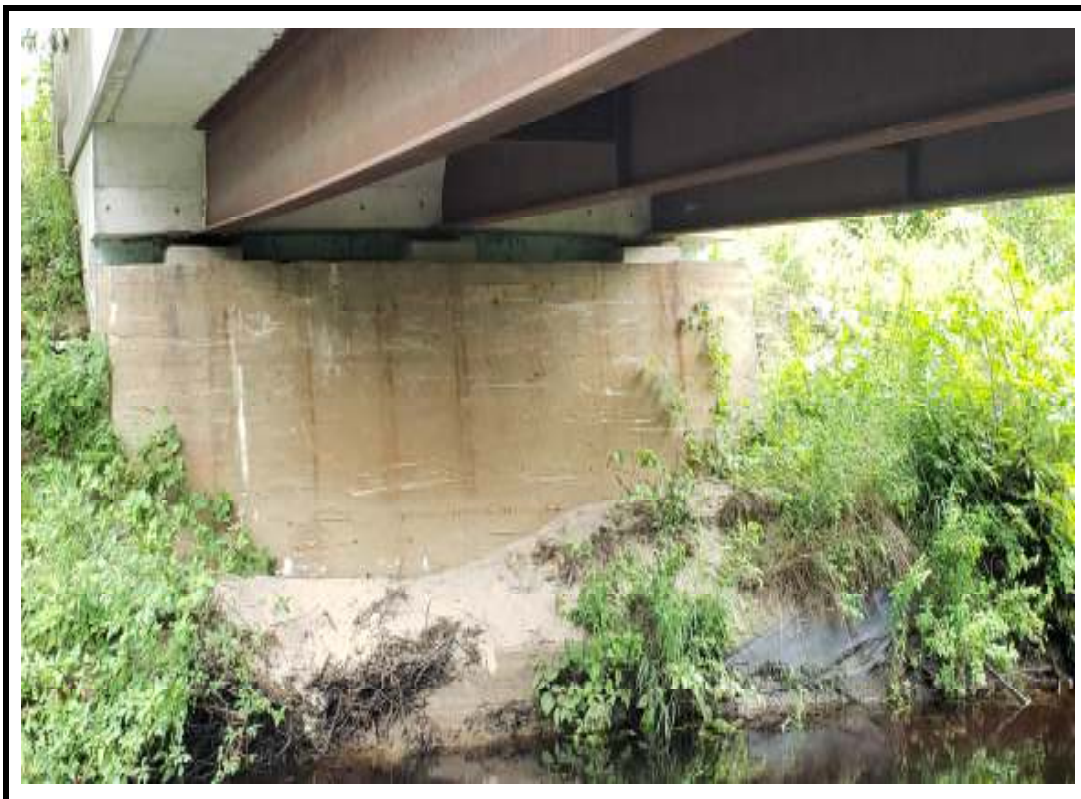
Photo 14 North abutment wall
