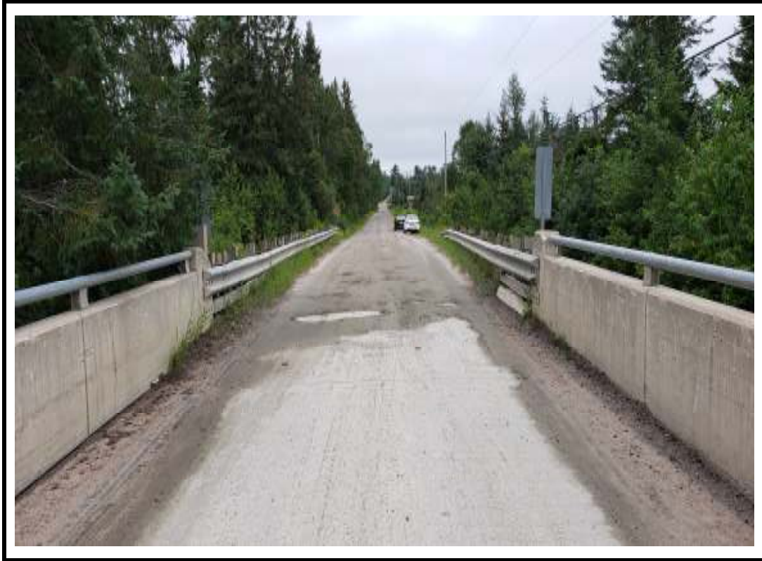
Photo 3 North approach from centre of structure
