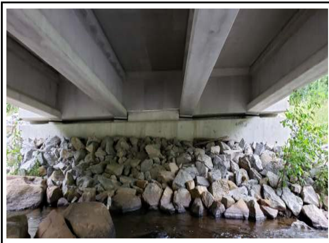
Photo 14 West abutment wall
