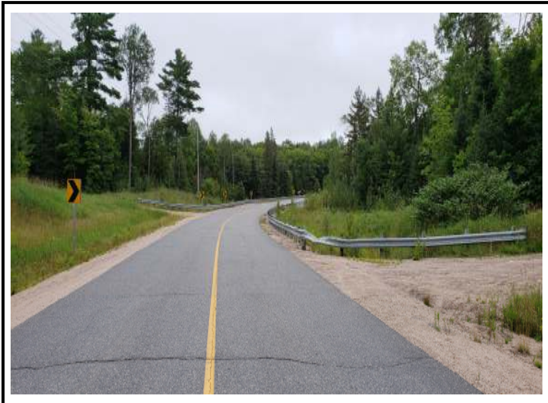
Photo 2 Structure from west approach
