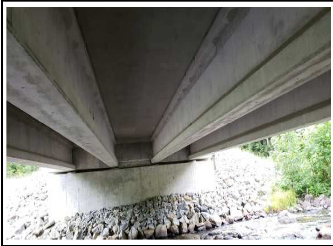
Photo 11 East underside of structure
