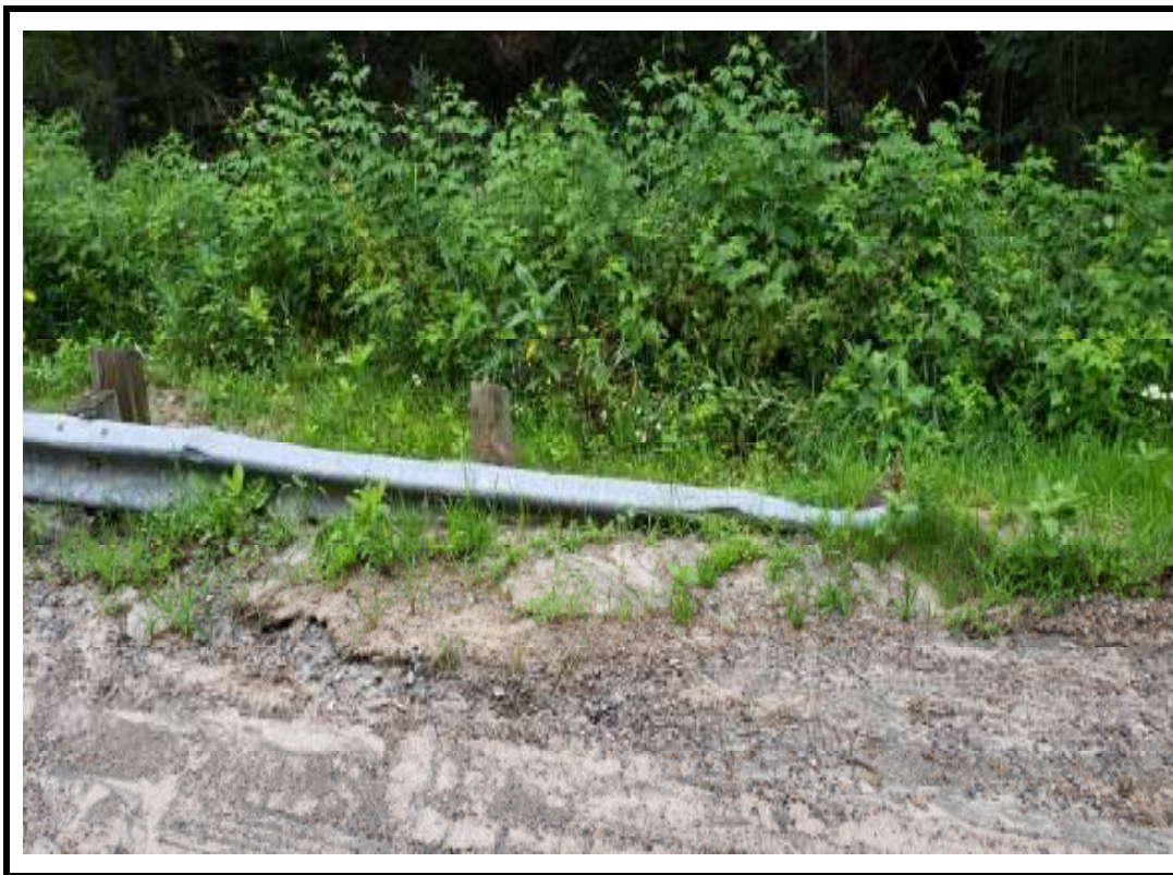
Photo 11 Southwest end treatment was buried into ground
