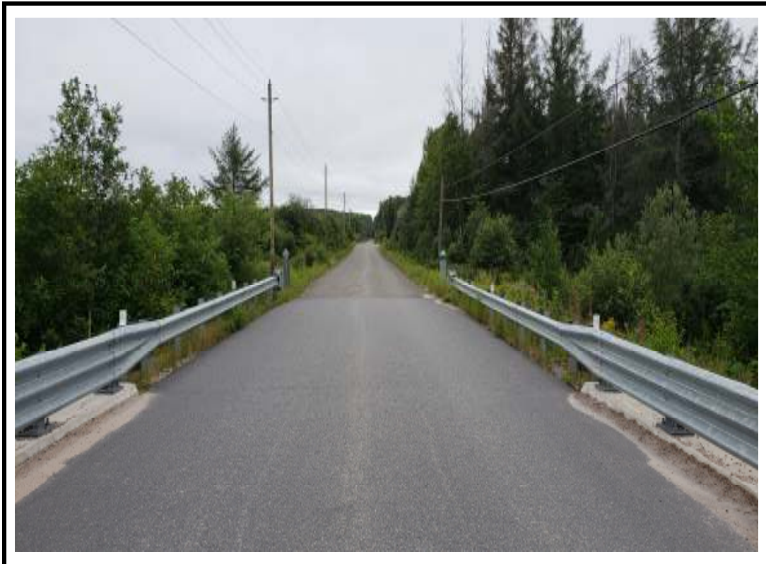
Photo 4 South approach from centre of structure
