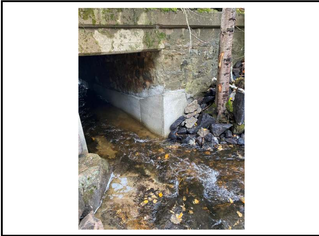
Photo 19 Southwest wingwall (after 2020 rehabilitation)
