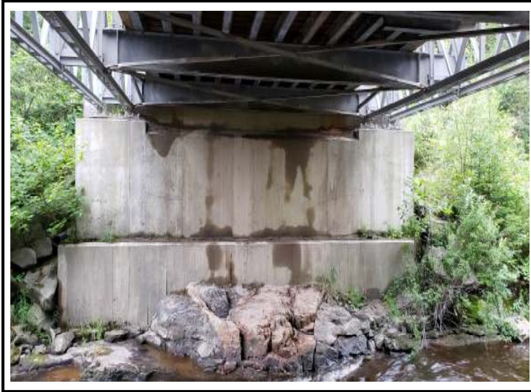
Photo 17 West abutment wall
