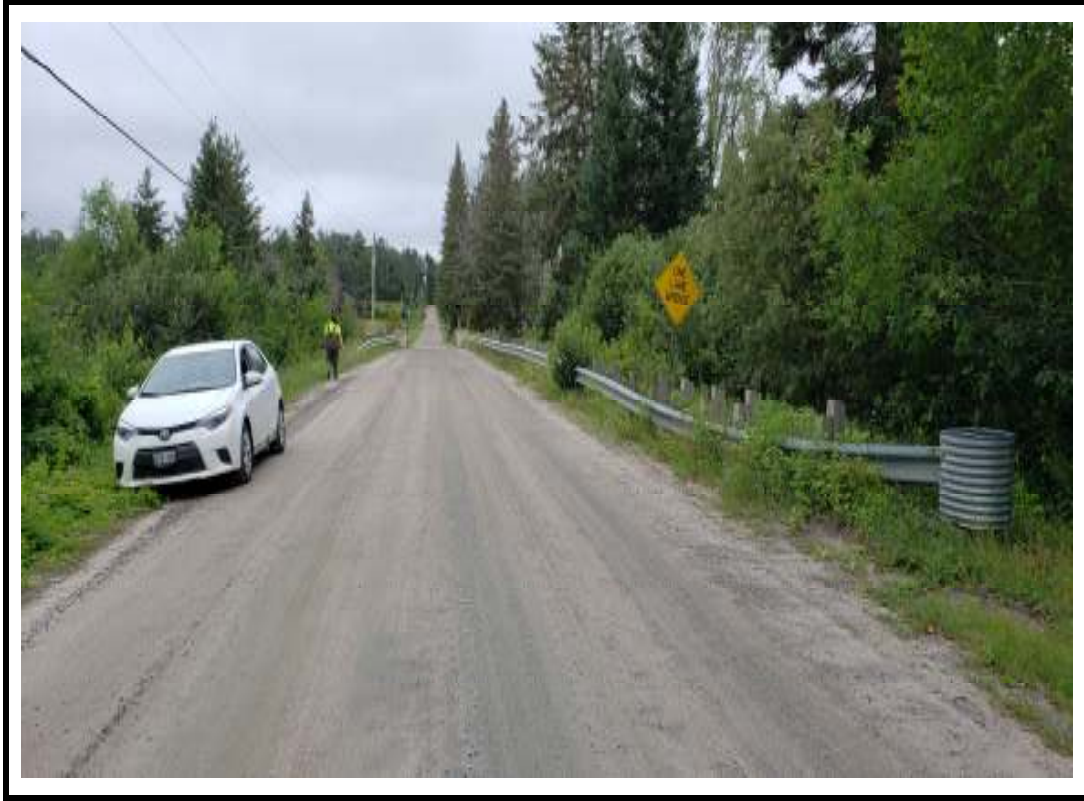
Photo 1 Structure from north approach
