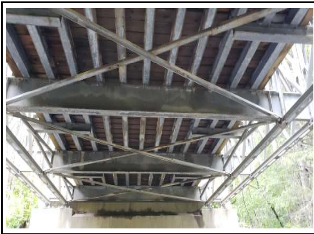
Photo 13 East underside of structure
