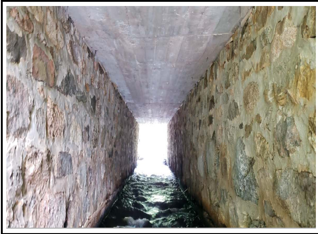
Photo 9 West underside of structure
