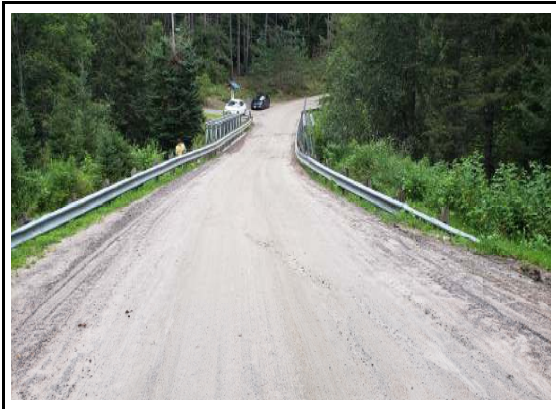
Photo 2 Structure from west approach
