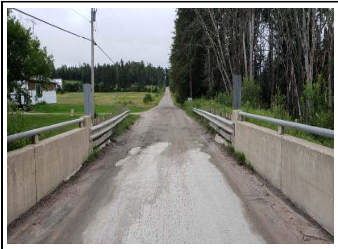
Photo 4 South approach from centre of structure
