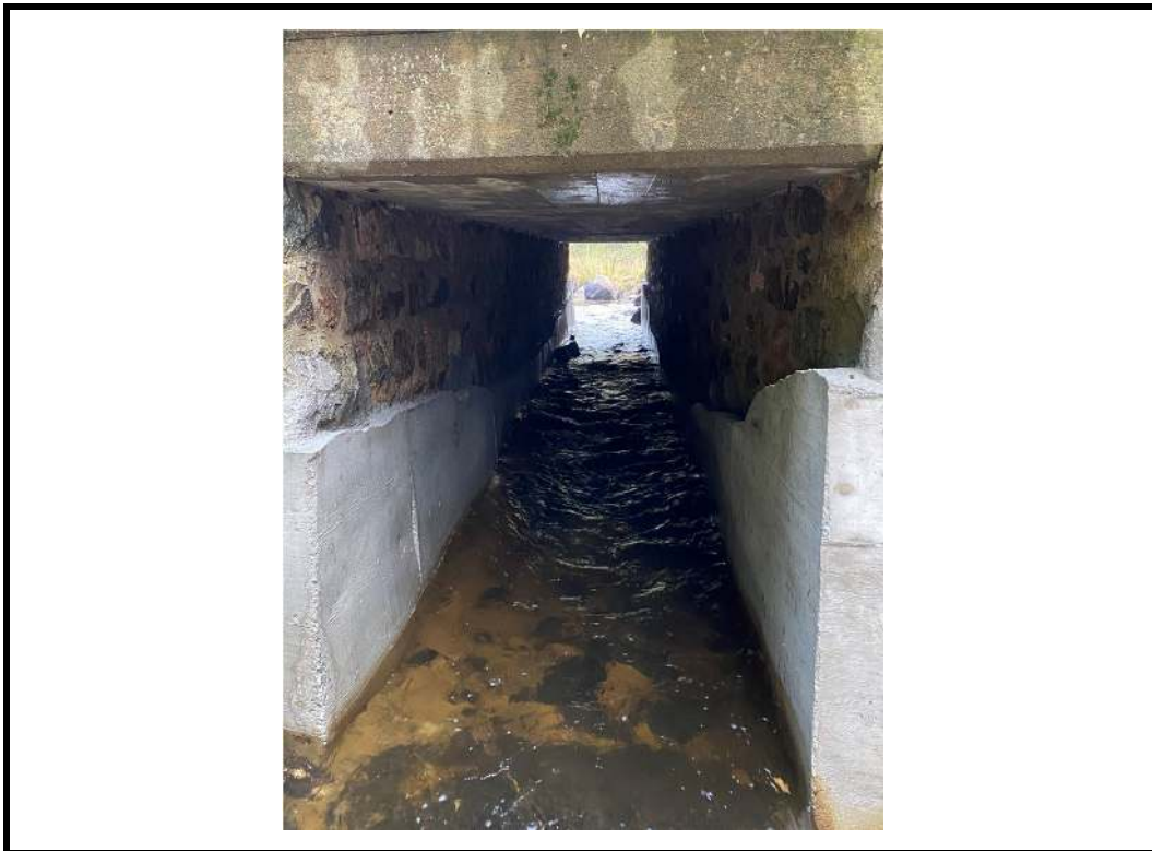
Photo 20 Barrel from east (after 2020 rehabilitation)
