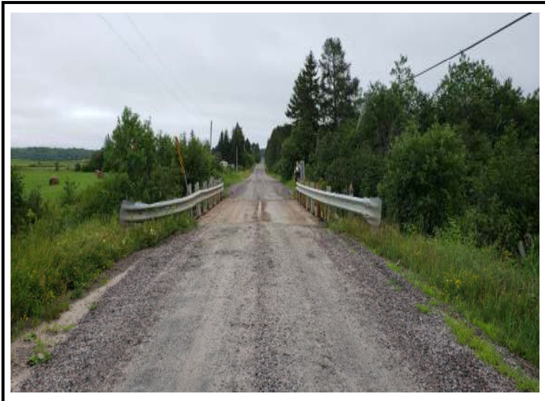
Photo 2 Structure from west approach
