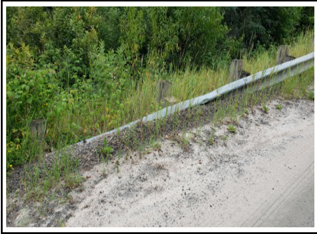
Photo 7 Northeast end treatment buried into ground
