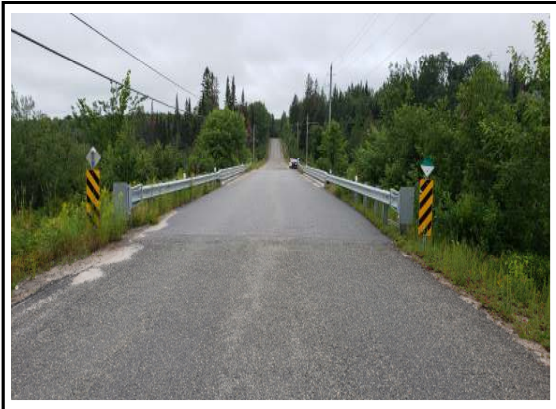
Photo 2 Structure from south approach
