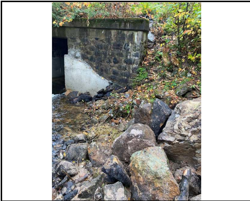
Photo 16 Northeast wingwall (after 2020 rehabilitation)
