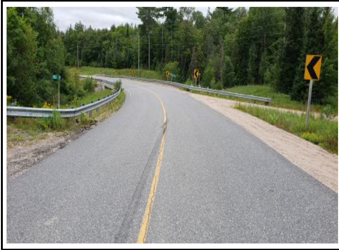
Photo 1 Structure from east approach
