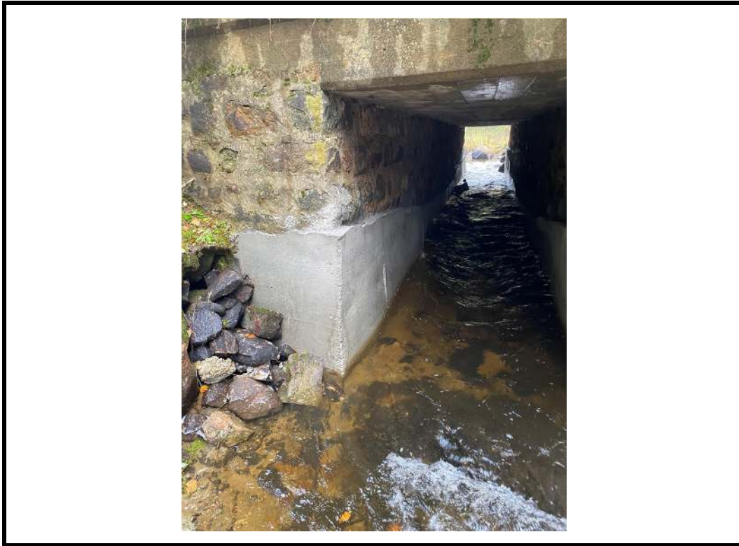
Photo 21 Southeast wingwall (after 2020 rehabilitation)
