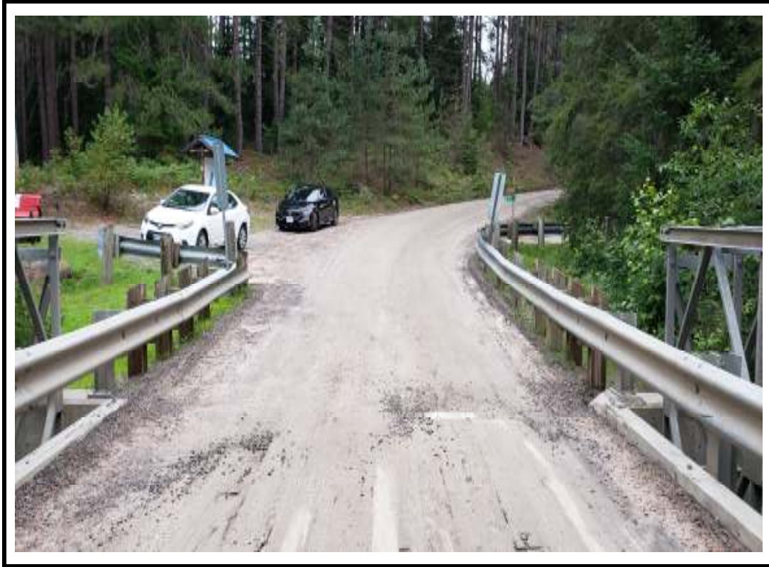
Photo 3 East approach from centre of structure
