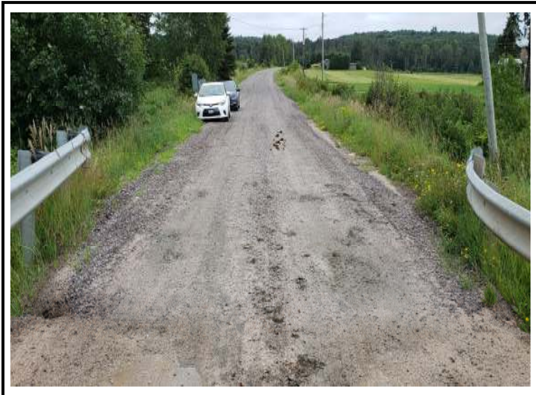
Photo 4 West approach from centre of structure
