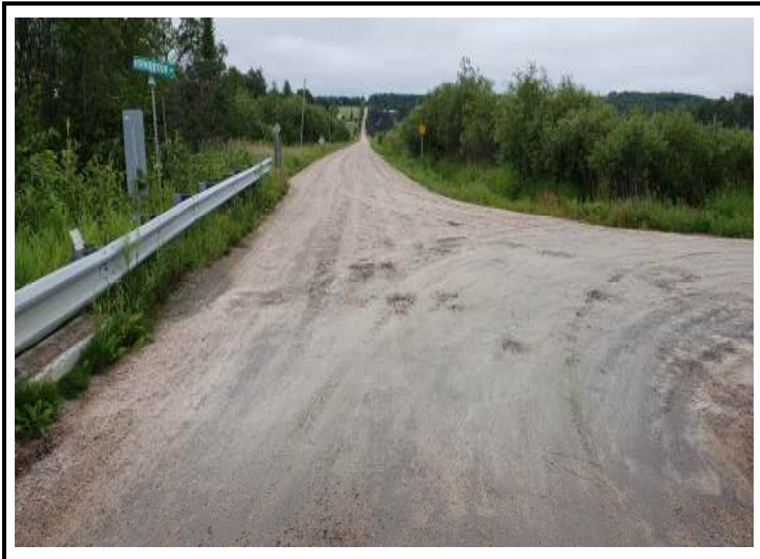
Photo 4 West approach from centre of structure
