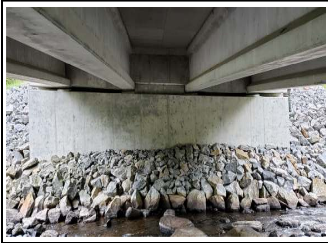
Photo 13 East abutment wall
