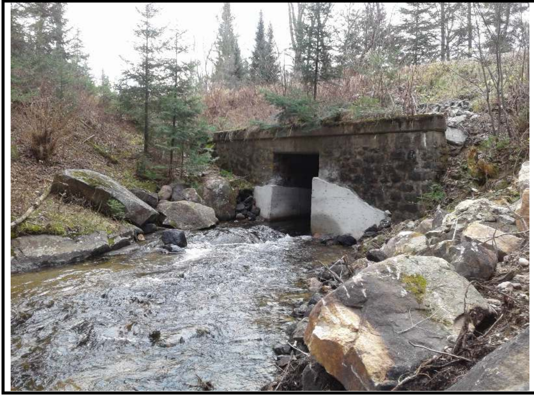
Photo 15 East Elevation (after 2020 rehabilitation)
