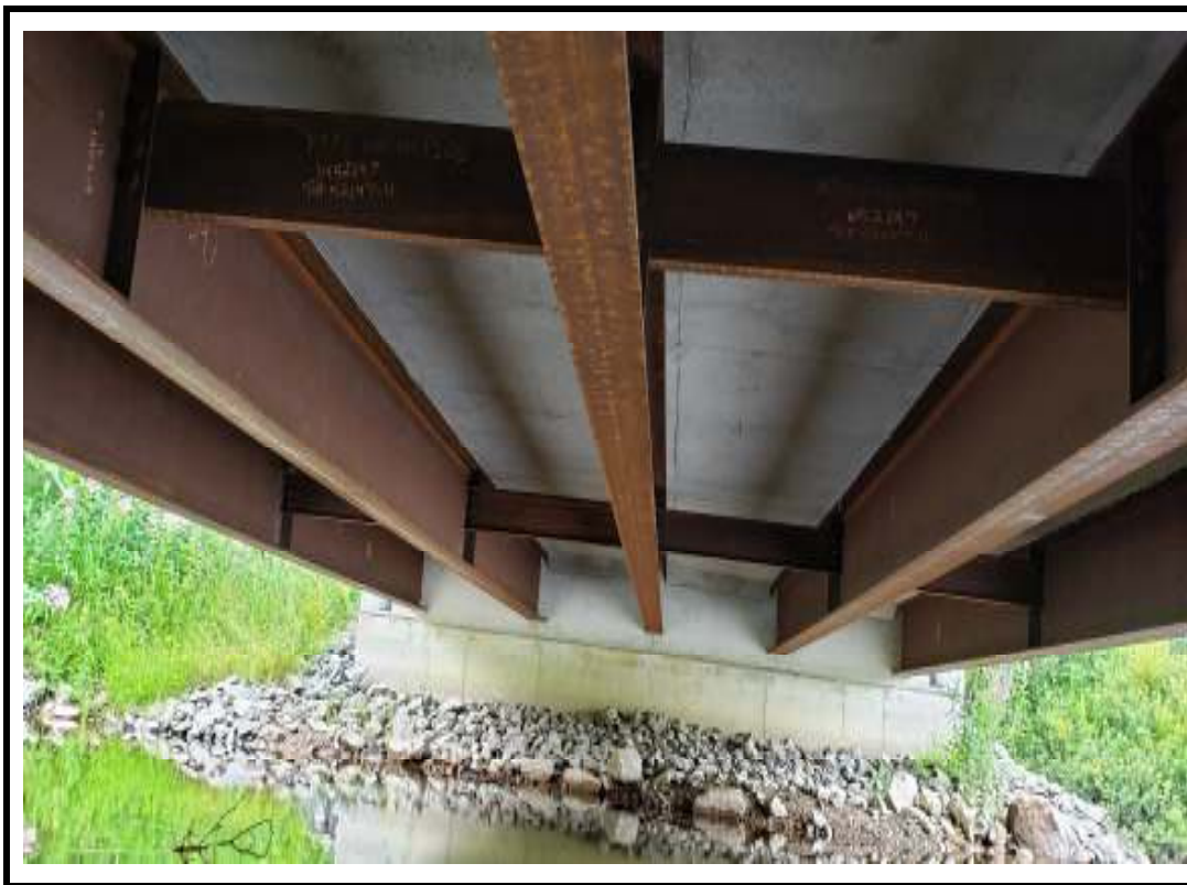
Photo 9 North underside of structure
