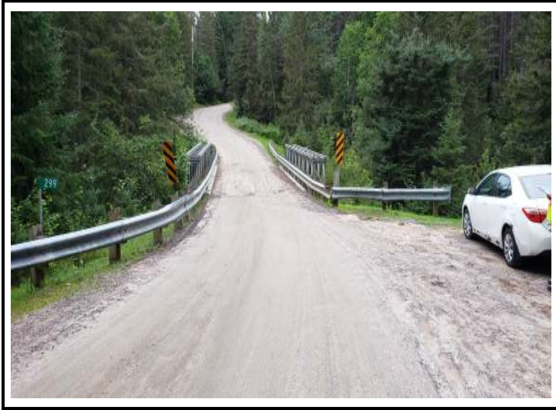
Photo 1 Structure from east approach
