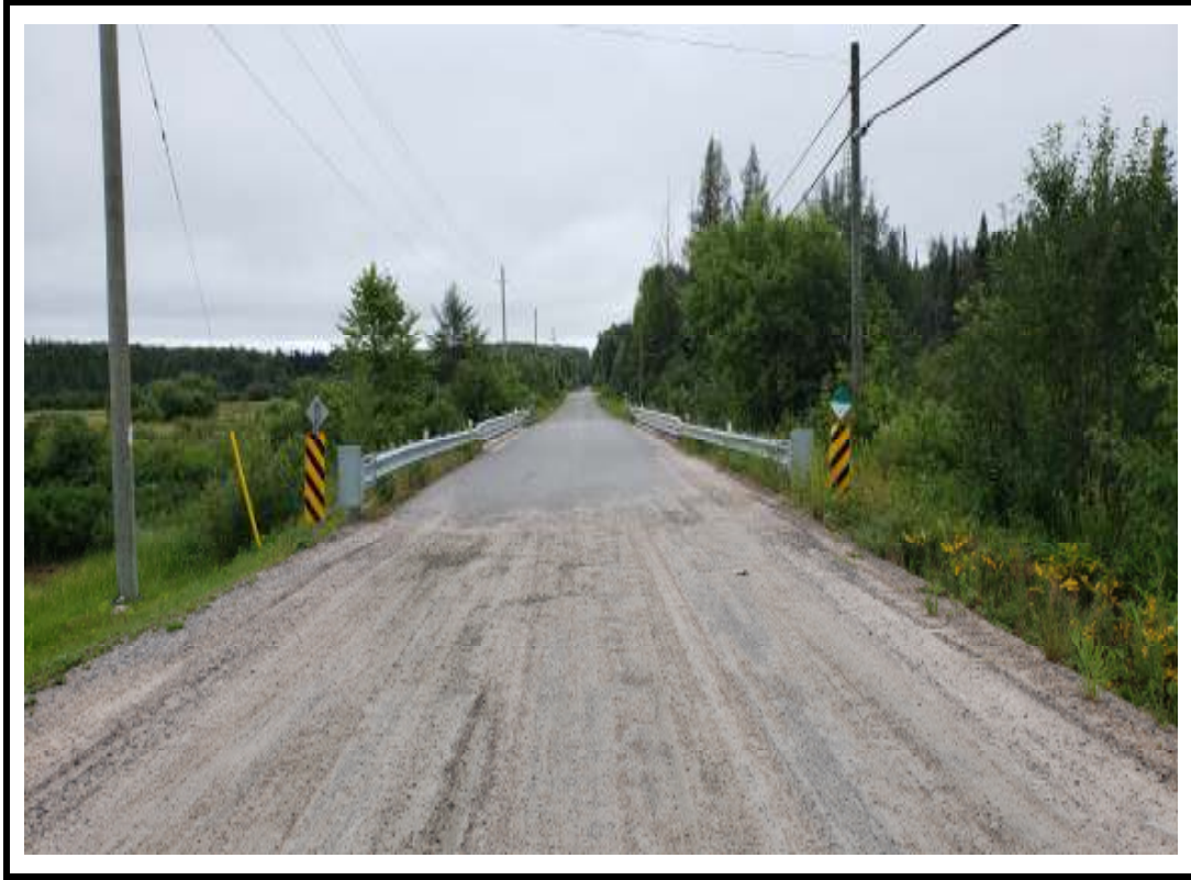
Photo 1 Structure from north approach
