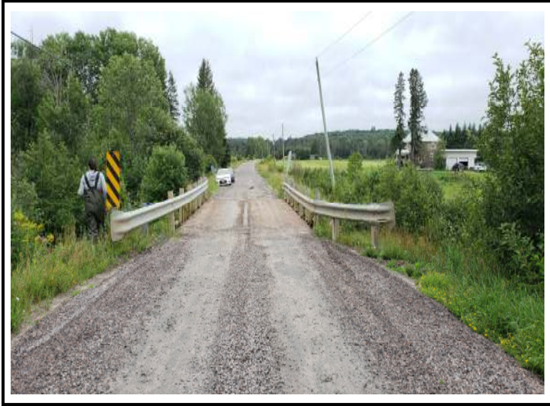
Photo 1 Structure from east approach
